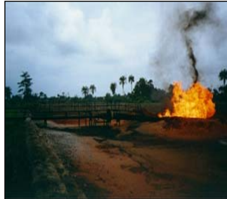
Appendix 4.4 Gas Flaring From Ruptured Pipeline
